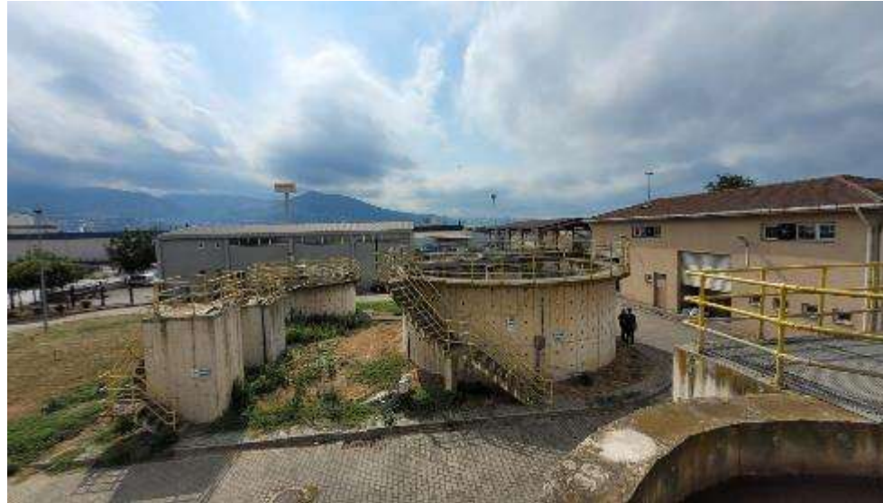
Figure 2-2: Overview of the WWTP
