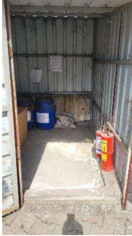
Figure 7-4: Temporary Storage Area for Hazardous Waste
